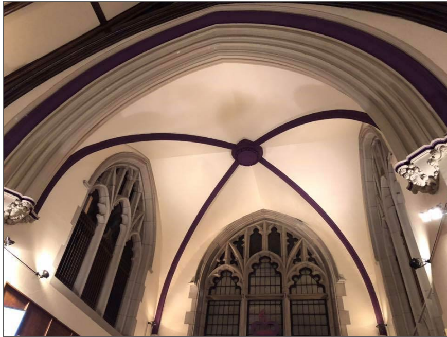
Sanctuary ceiling repairs and resurfacing 2018
