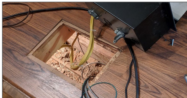
Stage box wiring and installation for new sound system, 2019
